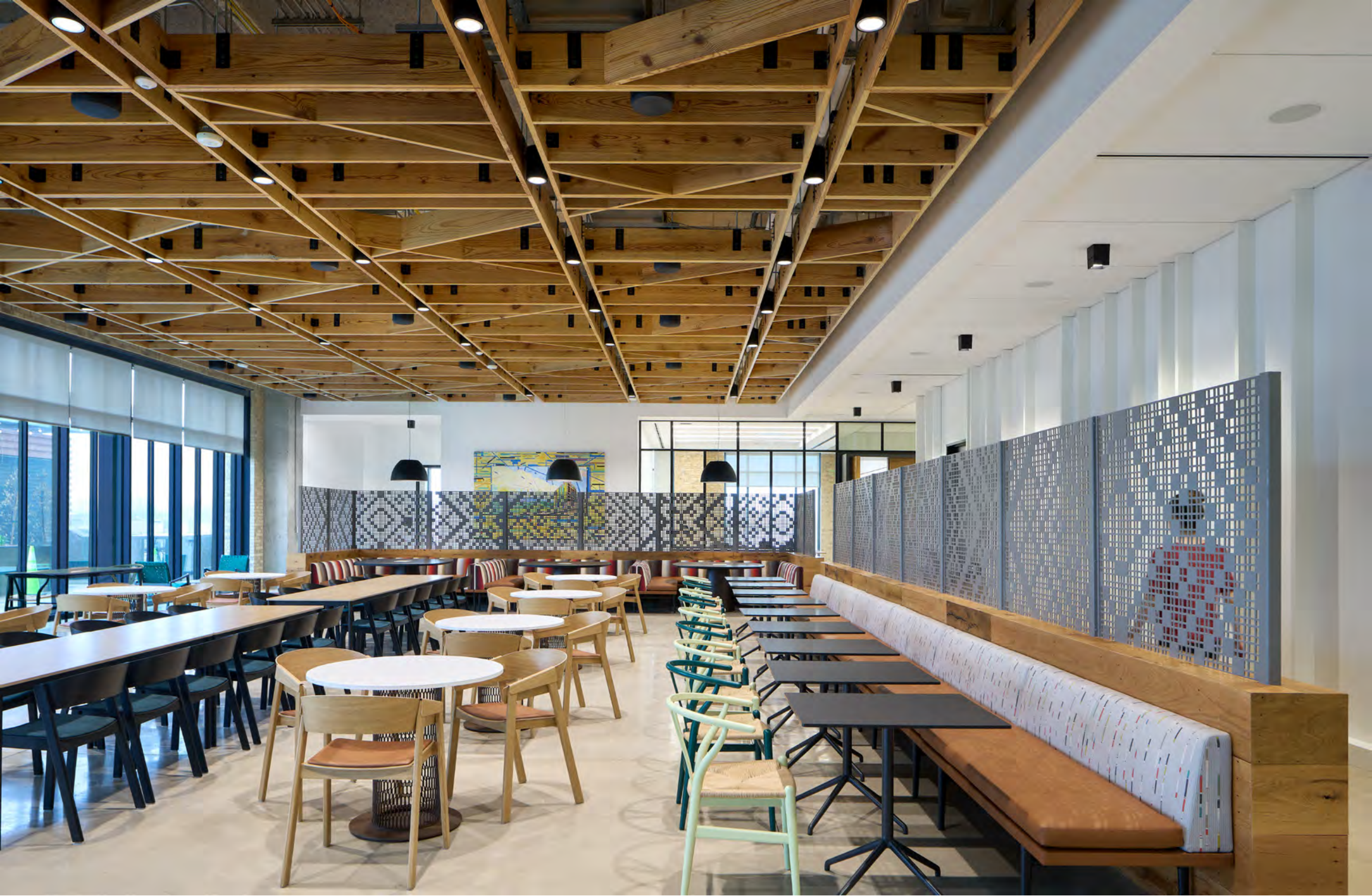
The biophilic trellis is made from reclaimed wood from the building demo, located 1.3 miles from the site. All artwork provided by local San Antonio artists.
